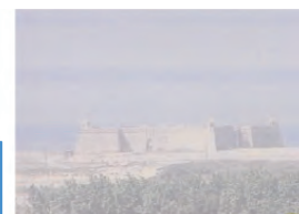
After two inch scratch repair
